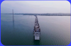
Mangla Dam 5 KM
